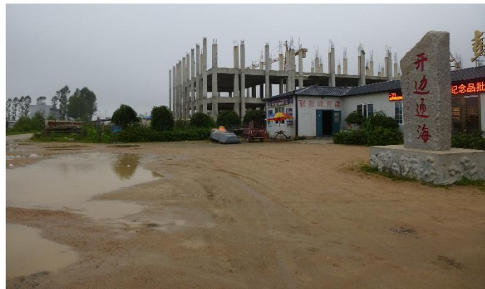
Figure 21: Construction Site at the Border Next to Border History Museum
