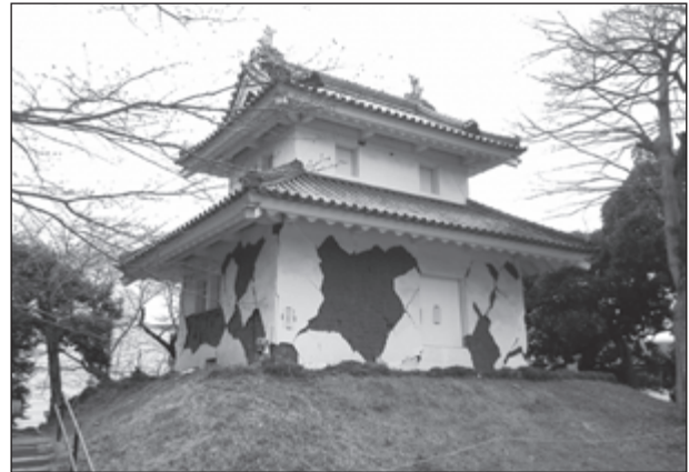
Figure 1. A historical building of Tsuchiura Castle (Ibaraki Prefecture) damaged by the Great East Japan Earthquake. Photo courtesy of Takachika Kimoto.
