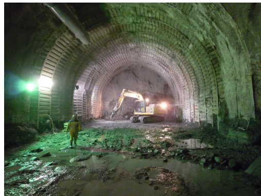
Figure 3.10: This picture shows civil works inside the near detector cavern. It is expected that the lab will be ready for detector installation in the middle of 2013 and ready for data taking early 2014.
