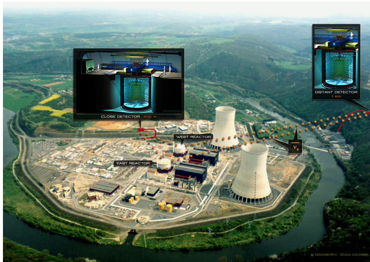
Figure 3.1: Surrounded by the meuse-river, on this aerial photography one can see the two nuclear reactors of the Chooz Nuclear Power Station. Added to this photography are the rough positions of the far and near detectors (labelled as close detector). Picture courtesy of CEA/IRFU.
