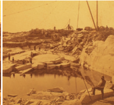
Abbildung 164: Eastern Point granite quarry, c. 1880, Stereograph, Cape Ann Museum Library & Archive, Gloucester (MA). Quelle: https://fitzhenrylaneonline.org/historical_material/?section=Granite+Quarrying+%2F+Shipping [09.09.2022].
