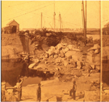
Abbildung 163: Eastern Point granite quarry, c. 1880, Stereograph, Cape Ann Museum Library & Archive, Gloucester (MA). Quelle: https://fitzhenrylaneonline.org/historical_material/?section=Granite+Quarrying+%2F+Shipping [09.09.2022].
