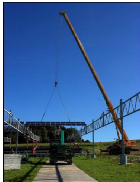
Fig. 5. (Right, source: farm community Heggelbach): Installation of APV power plant with mobile soil protection panels in August 2016.
