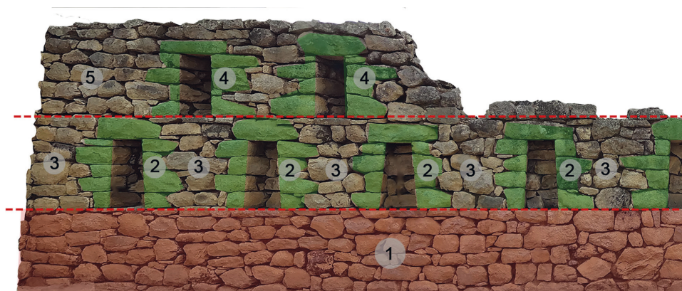
Figure 1. The wall of Kallanka (Sector 5D) with construction phases, orthoimage.
