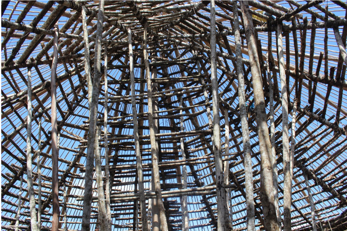
Figure 18. Scaffolding structure used in the construction of the ättä (Pablo Albernaz)
