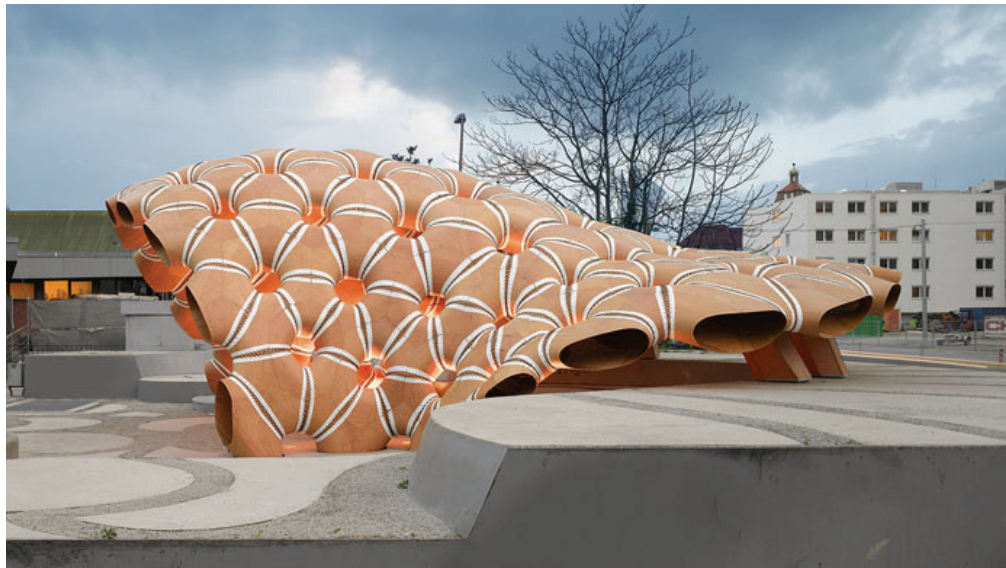
Fig. 11.12 ICD/ITKE Research Pavilion 2015. The front view showing the transition from shell to plate-and-pillar system (Photo: Roland Halbe)
