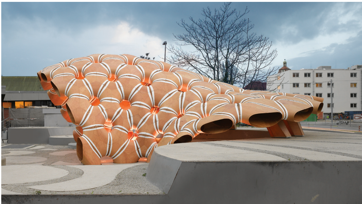
Figure 39. ICD / ITKE Research Pavilion 2015 at the University of Stuttgart. Developed during an interdisciplinary biomimetic course together with the University of Tübingen. From Grun et al. (2016)
