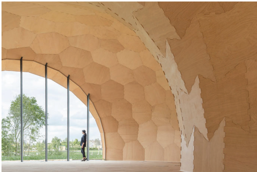
Fig. 11.6 Landesgartenschau Exhibition Hall in Schwäbisch Gmünd, Germany. Interior view showing the polygonal plate layout of the single-layered segmented shell (Krieg et al. 2015)
