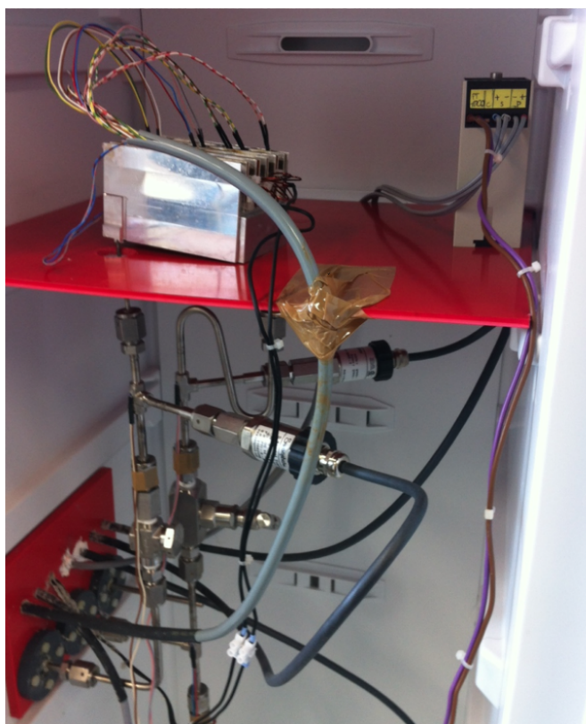
Figure 6.22.: The interior of the thermal insulation enclosure.
