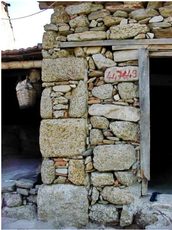
Abb. 60: Kapıkırı, Haus 63, Mauerdetail
